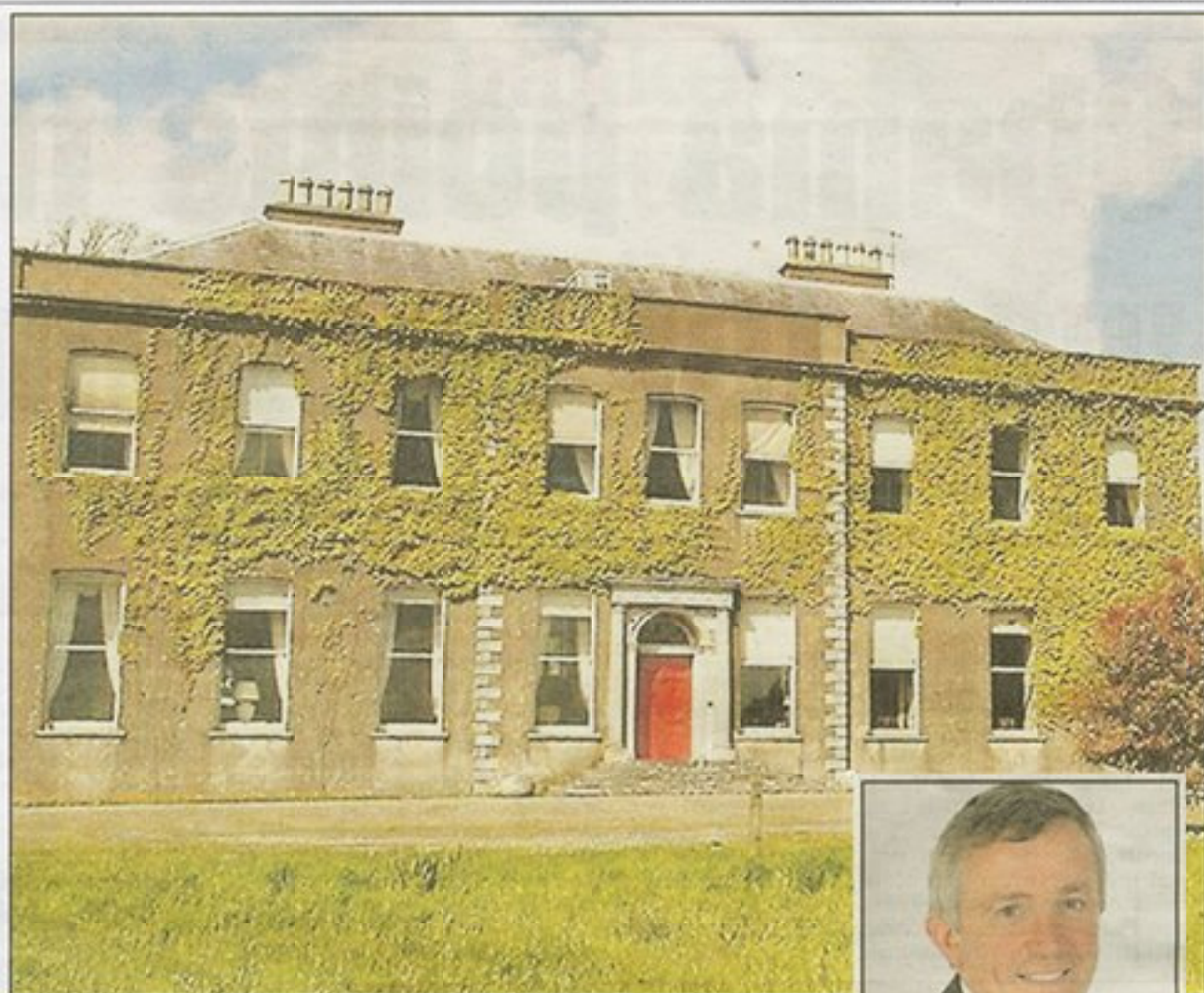
Dunkettle House, above, which will be restored to its former glory as part of the €400m development of the site and right: Michael O'Flynn, managing director of O'Flynn Construction who are carrying out the project.
